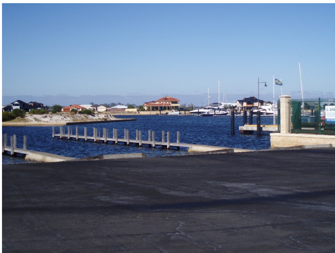
Canal development at Port Geographe, WA, as inspected by Committee members
